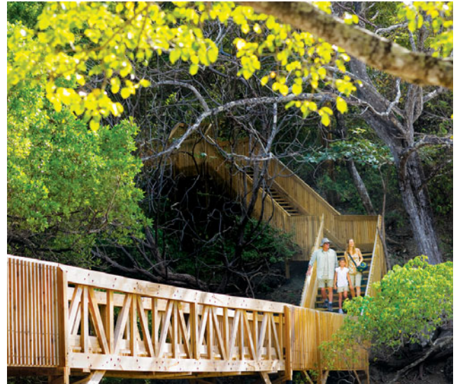
Wooden Stair System at Peninsula Papagayo
